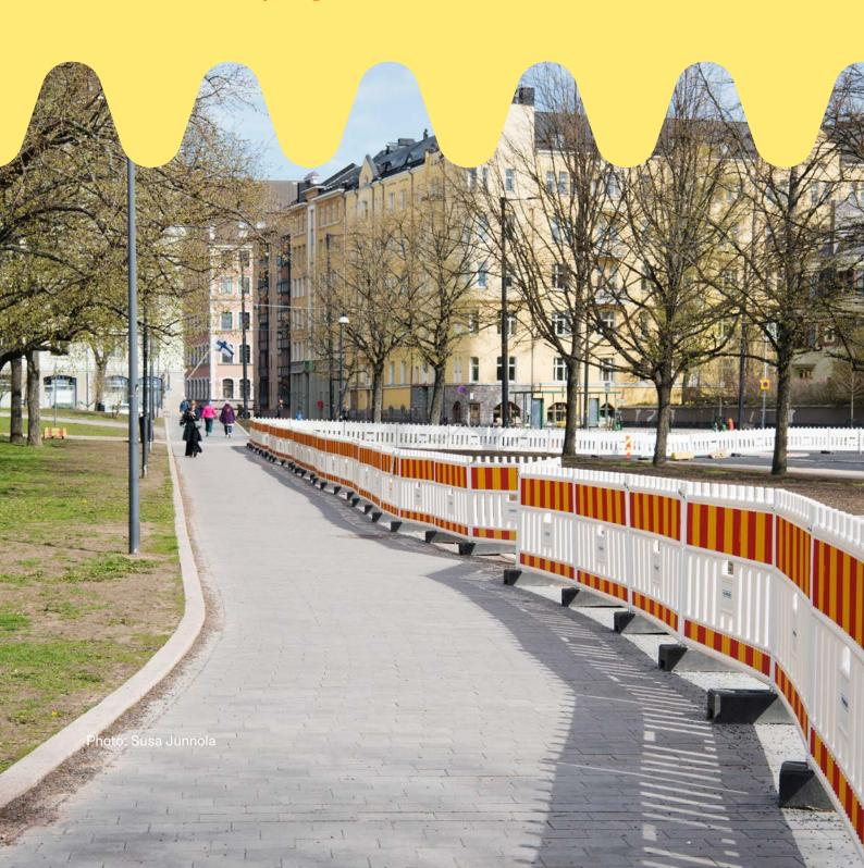
This means the appropriate consideration of route width, worksite fences, route sloping, and the materials and maintenance of route surfaces, among other things. This way, it can be ensured that people using a wheelchair or walking with a pram can easily traverse the route from start to finish.
